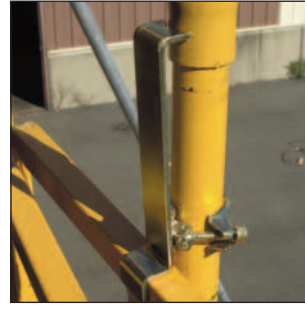
Rotation blocking ring of the brace
